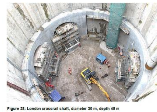
Figure 28: London crossrail shaft, diameter 30 m, depth 45 m
